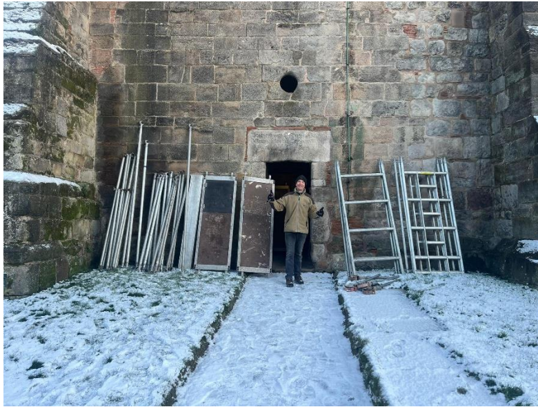
Scaffolding ready to carry up the tower
